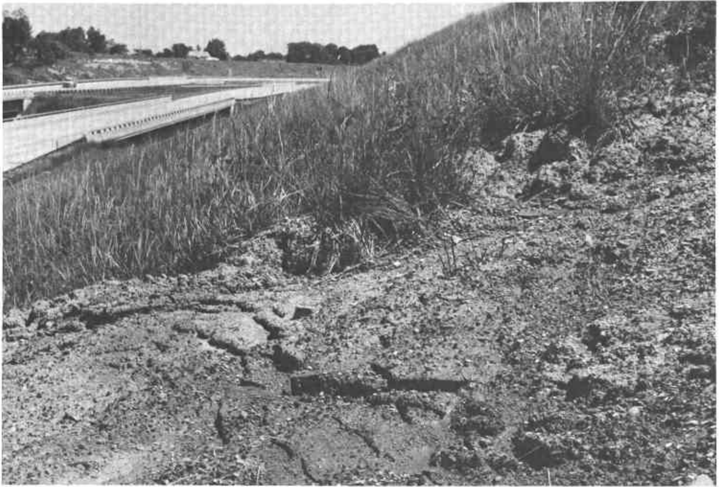
Figure 5.—Soil slip along road cut. Seepage areas in the substratum of Haskins soils result in instability.
