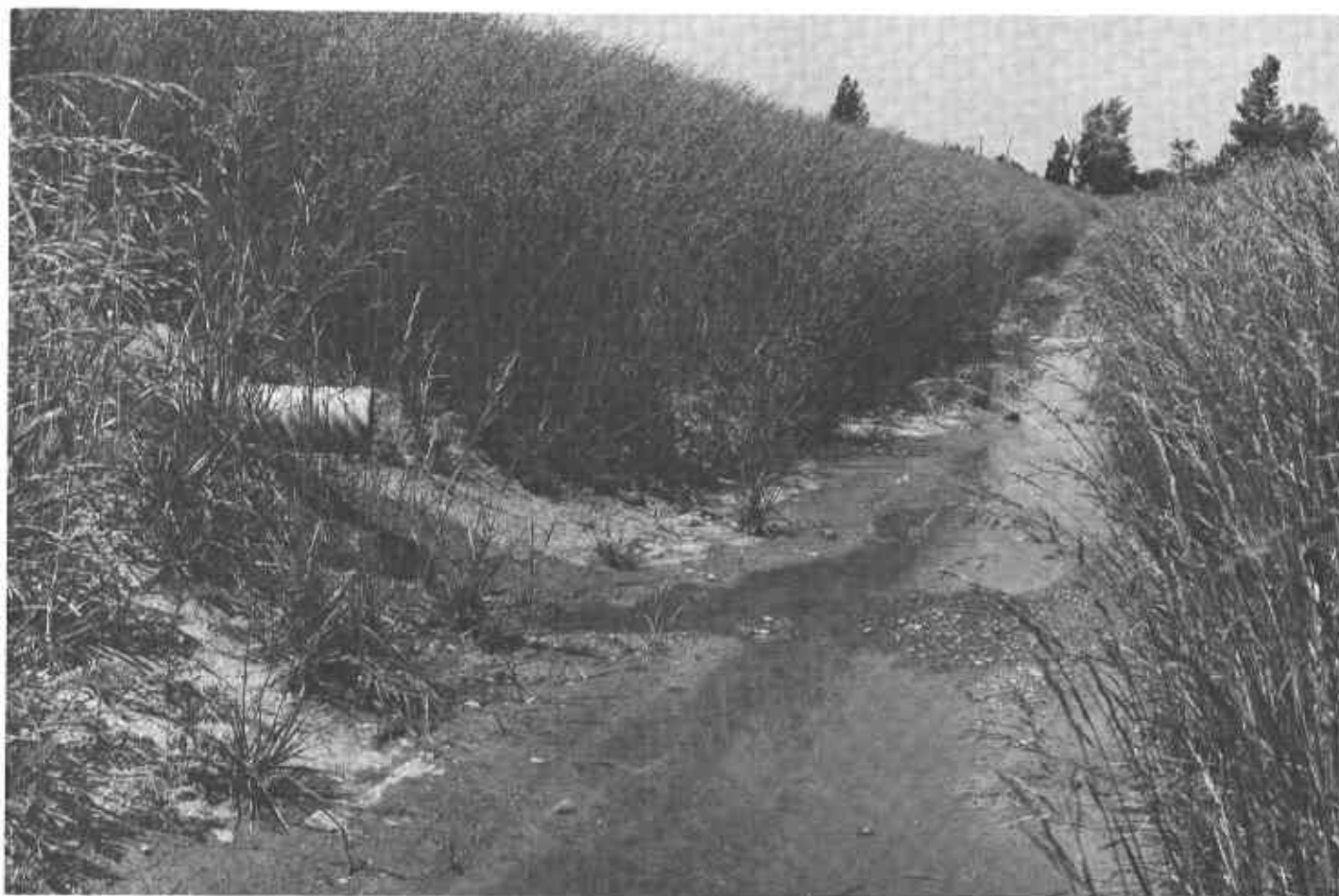
Figure 6. —Drainage ditch in a Mahoning silt loam. Outlet pipes for tile and grassed slopes minimize erosion and maintenance of this ditch.
