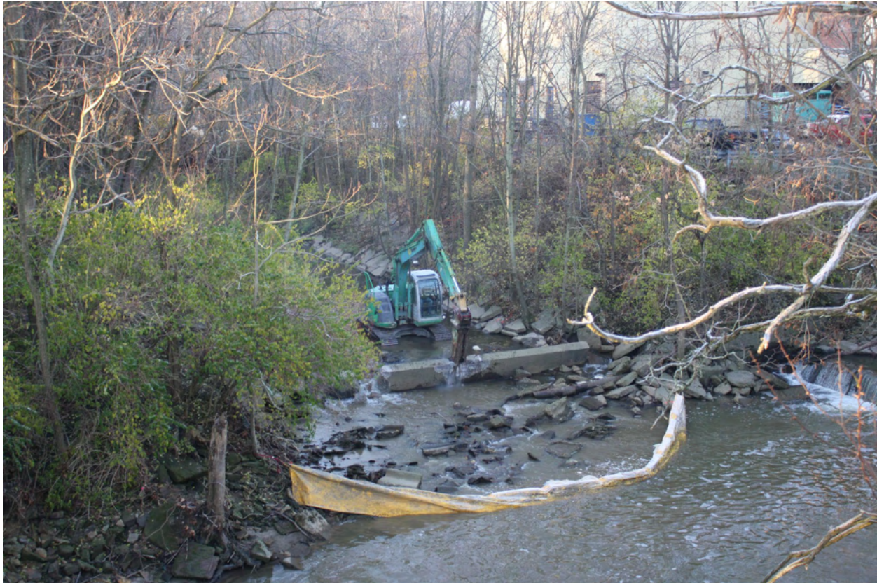
Low head dam removal.
