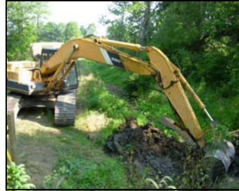
Schroeder Ditch Project—Phase II
